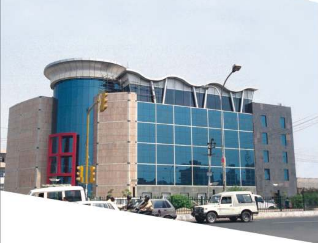
Sab Mall, Noida Building enclosure in steel with a working height of about 20 mtrs.
