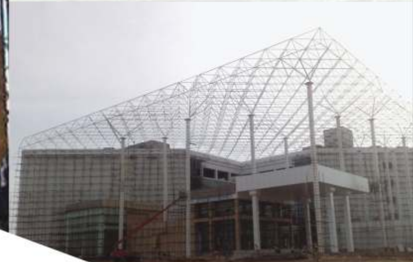
Geodesic dome - KIPT, Bhubhaneshwar A state-of-the-art design of Geodesic spaceframe structure with glass cladding.
