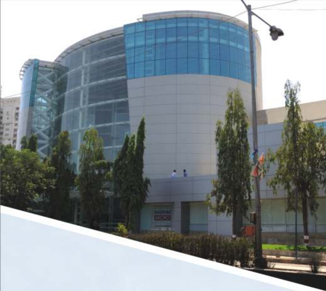
K-Park, Mumbai This elliptical standalone Steel Atrium has a 24 mtrs. working height and extends over 21 mtrs. of area.
